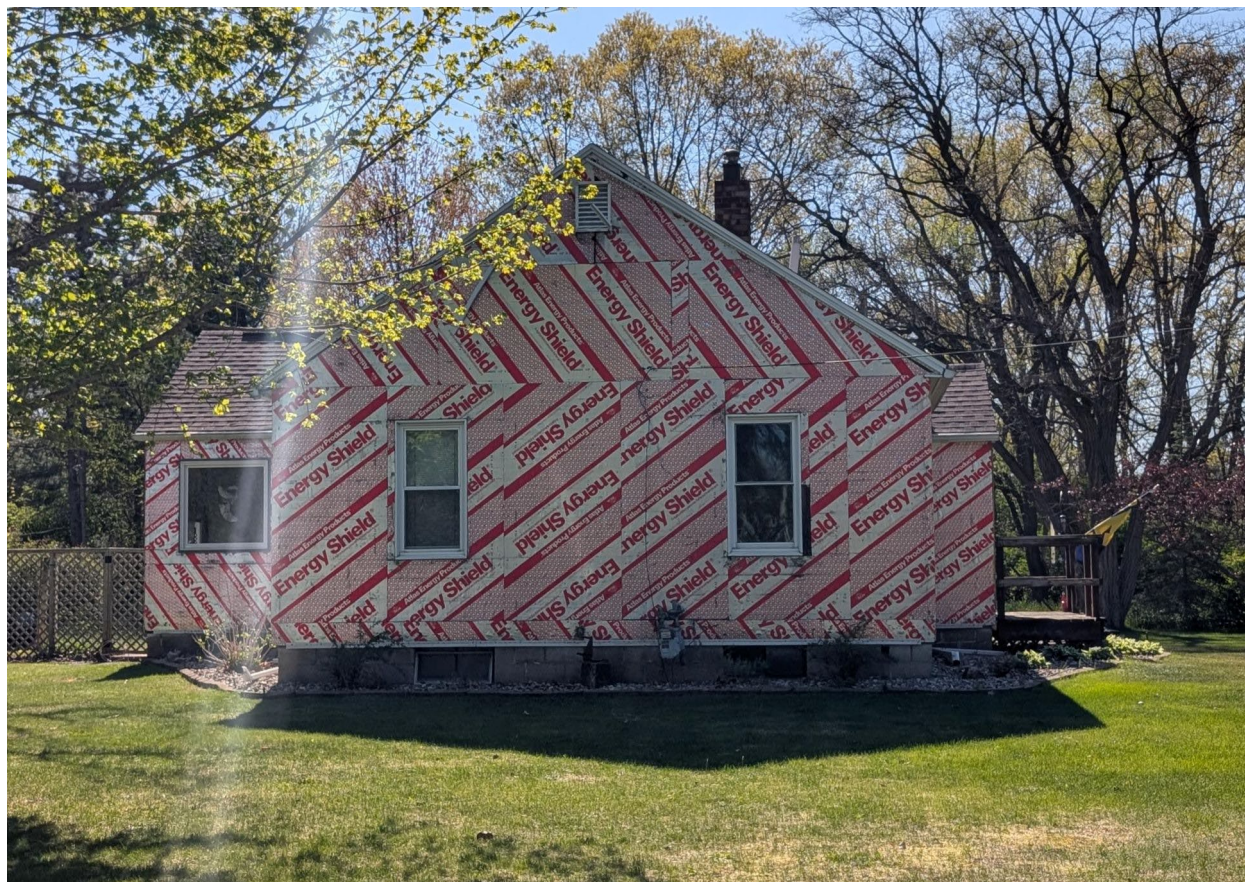
[EnergyShield® being re-used during siding replacement, photo courtesy of ATLAS]
