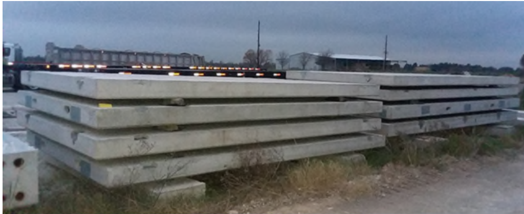
Typical Wall Panels in Storage
