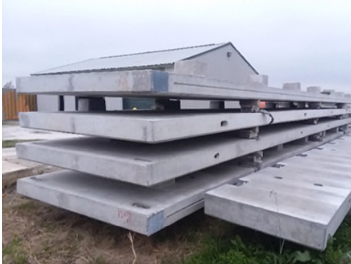
Typical Spandrel Panels in Storage
