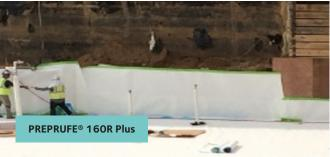
PREPRUFE® Plus membranes are release liner free and designed for efficient, reliable installation. PREPRUFE® Plus ZipLap™ seams allow for an adhesive to adhesive bond at membrane sheet overlaps and deliver superior performance in harsh conditions without the need for specialized equipment, heat or power.
